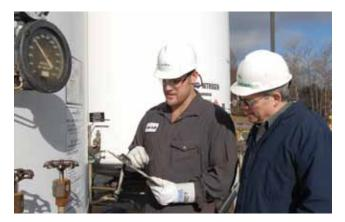
▲ Figure 1. Gaseous nitrogen, vaporized from onsite liquid storage into a local distribution system, is used for a wide variety of applications, including blanketing, inerting, purging, stripping, and sparging. Other supply modes ranging from cylinders to onsite generation are also used to deliver nitrogen gas.
